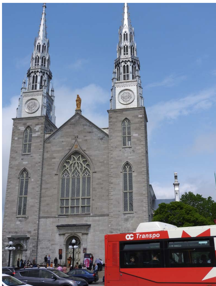
This Notre Dame Basilica and one-time La Salle Academy, a French Catholic institution, had an Irish Catholic counterpart just down the street, not an infrequent juxtaposition.
