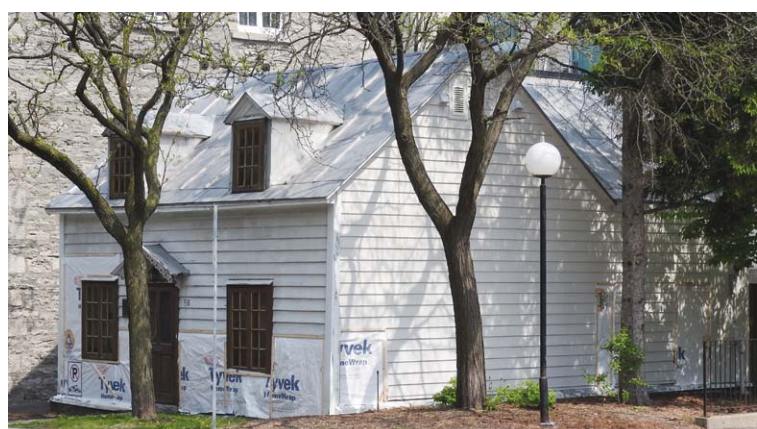
Tin House Court is a tourist destination in Ottawa, featuring this reconstructed building in an area where wooden homes were forbidden. It was a metal exterior covering a log cabin.
